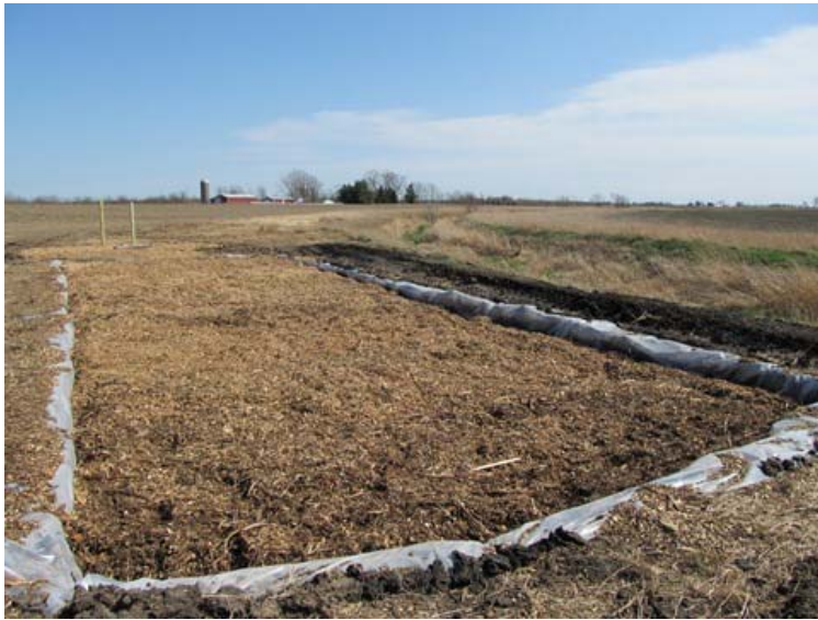
Wood chip bioreactor on a tile line draining 50 acres. Mark David
