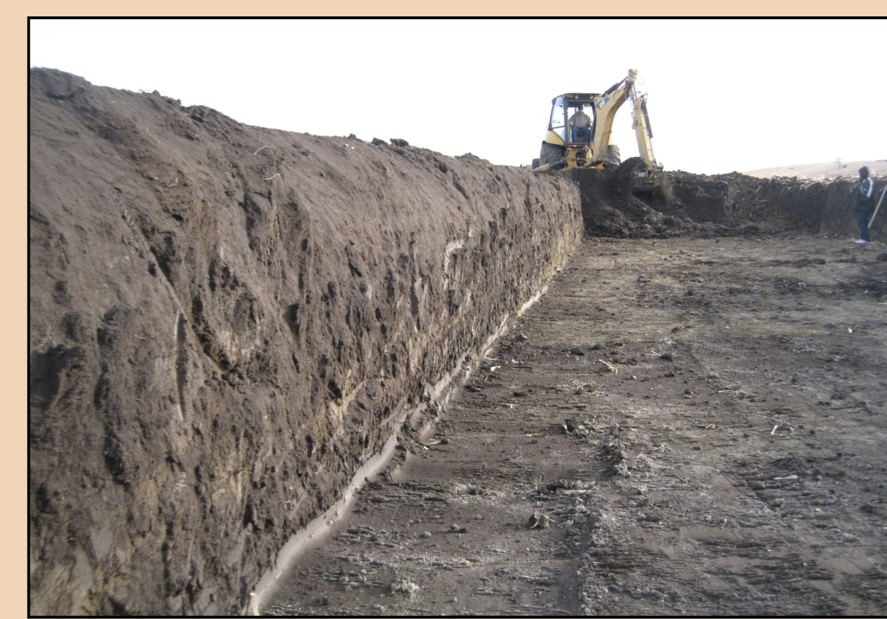
1. Excavating the trench about 21 ft. wide, 130 ft. long and 5 ft. deep for the bioreactor.
