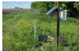
2011 spring after installation
