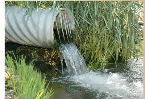
Figure 1. Subsurface tile drain outlet (courtesy of the Leopold Center for Sustainable Agriculture, Jerry DeWitt)
